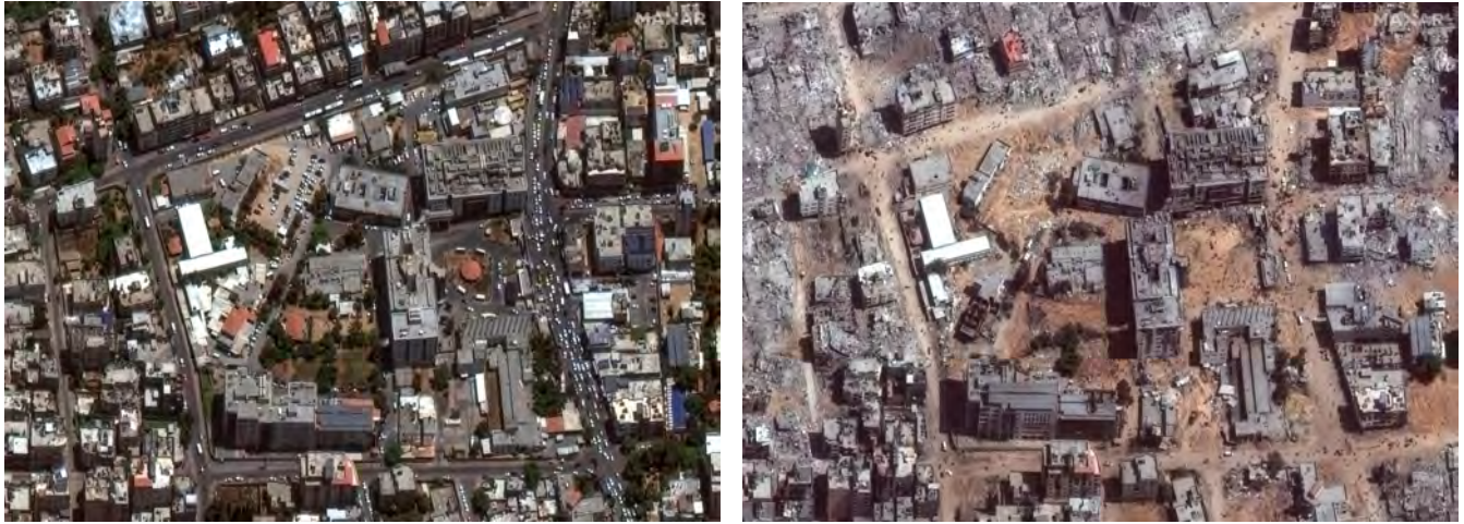
Figure 8. Al-Shifa Hospital Complex, before (left, 2022) and after (right, 2024). Satellite image from Maxar Technologies.
